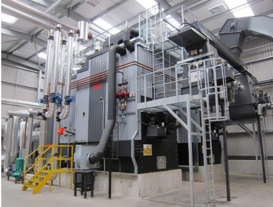
6MW Wood Chip Boiler at Sawmill Site in Mid-Wales, Photo Courtesy of Sustainable Energy Ltd
