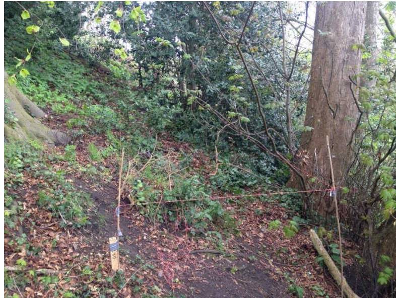
Photo 2 – Looking north near T89 showing boardwalk being located so as not to affect tree (Sycamore visible to the right of the picture). String line represents pegs 7 & 8 on setting out plan (Annex B).
