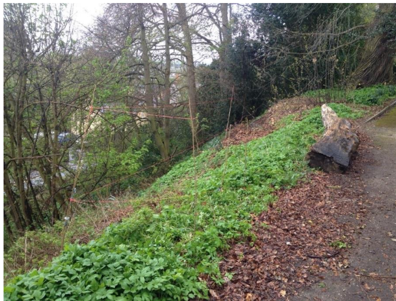
Photo 3 – Looking south from top of proposed boardwalk where it emerges onto the path. Lower string line represents deck level at pegs 1 & 2, with upper string line at 1.1m (suggested handrail height).
